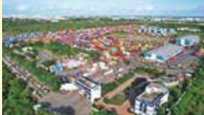
67 terminals Including 16 MMLPs setup across the country
